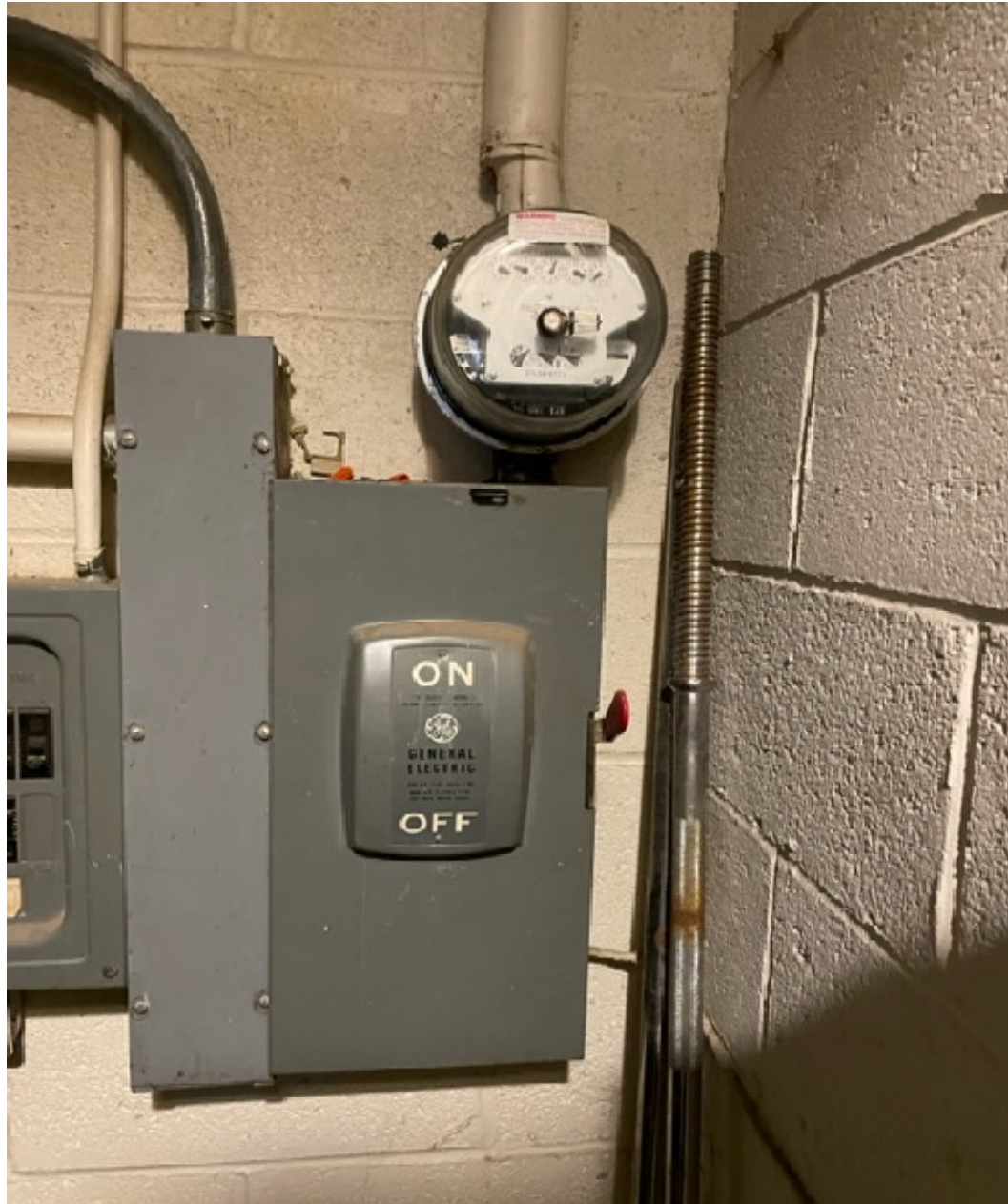
Photo 4 – Field House Electric Utility Service Meter and Disconnect
